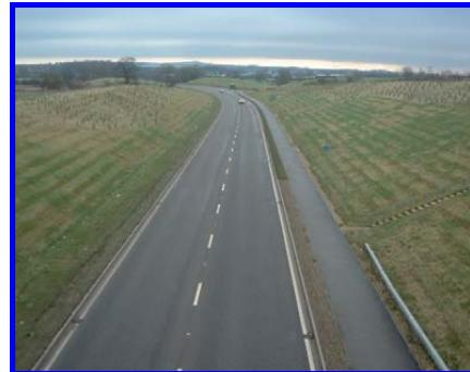
Part of the road intended for the movement of road motor vehicles; the parts of the road which form a shoulder for the lower or upper layers of the road surface are not part of the roadway, nor are those parts of the road intended for the circulation of road vehicles which are not selfpropelled or for the parking of vehicles even if, in case of danger, they may occasionally be used for the passage of motor vehicles. The width of a carriageway is measured perpendicularly to the axis of the road.
