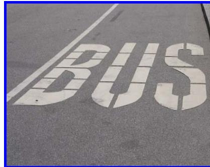
Part of a carriageway designated for buses and distinguished from the rest of the carriageway by longitudinal road markings.
