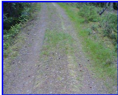
Road with a stabilized base not surfaced with crushed stone, hydrocarbon binder or bituminized agents, concrete or cobblestone.
