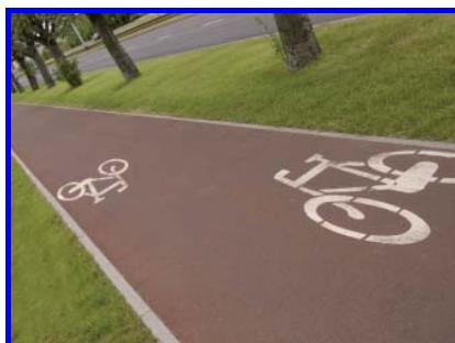
Independent road or part of a road designated for cycles and sign-posted as such. A cycle track is separated from other roads or other parts of the same road by structural means.
