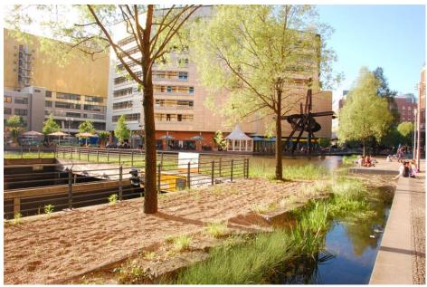
Picture 1: Open rainwater canals and bioretention pond in settlement (author: Zuzana Hudekova)
